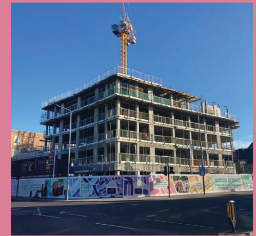
Figure 44: Families and Homes Hub Construction
