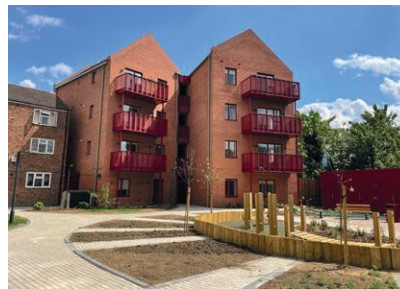
Figure 29: New Homes at Essex Close
